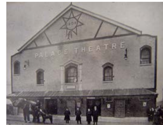
Below: the original Watford Palace Theatre building built in 1908.
